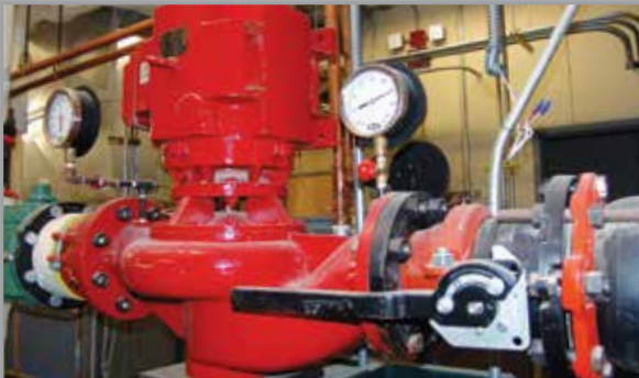
Woolworth Building —EnviroFlo Close-Coupled Vertical In-Line Pumps are providing world-class quality and reliability as they circulate condenser water to 18 units on three floors of this world-renowned structure in NYC.
